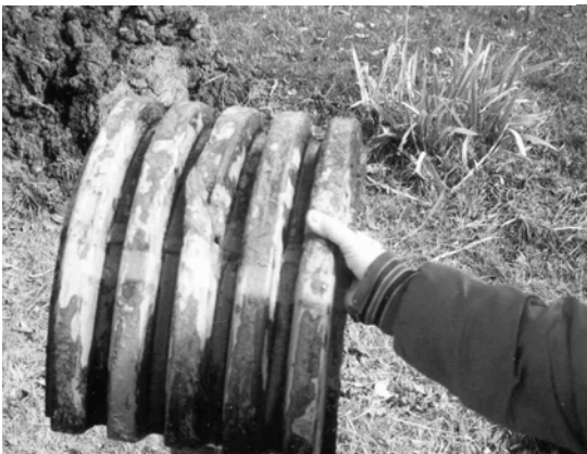
Figure 2 Pipe Cut Location
