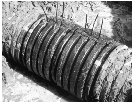
Figure 3 Split Band Installation
