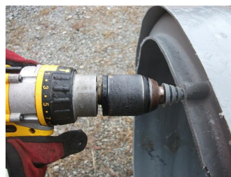
Figure 8: Holding Drill Flush
