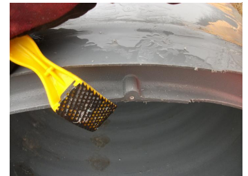
Figure 10: Finishing the Weld
